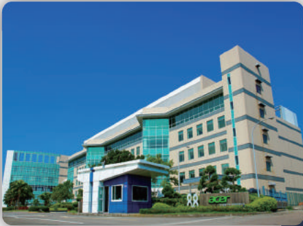
Data Center Hi-Tech Industry
